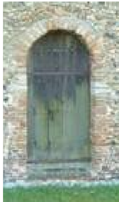
Roman brick in Mt Bures church door demonstrates the proximity of a Roman building of villa status, even though its exact site is unknown
